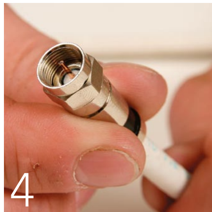
4 Slip the fitting over the stripped cable until it's flush with the receiving end.
